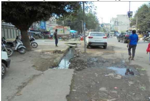
Figure 7-6: Open Drain, Kashipur Bypass Road
