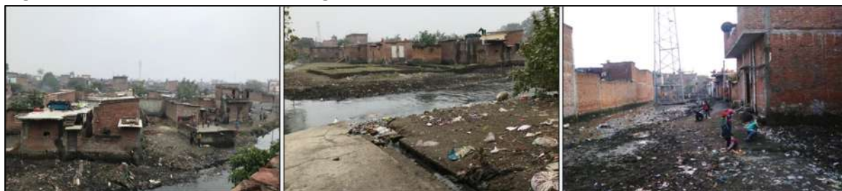
Figure 6-5 Slum Encroachment Along the Drains
