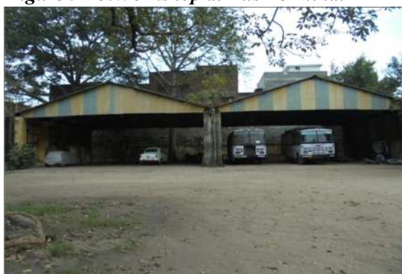
Figure 9-15: Workshop at Bus Terminal
