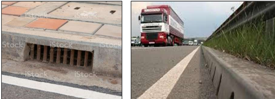
Figure 7-8 Storm water drainage illustration
