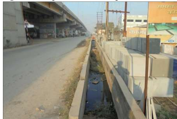
Figure 7-7: Open Drain, Kashipur Road
