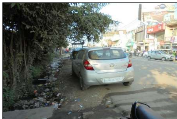
Figure 7-3: Open drain, Ramnagar Road
