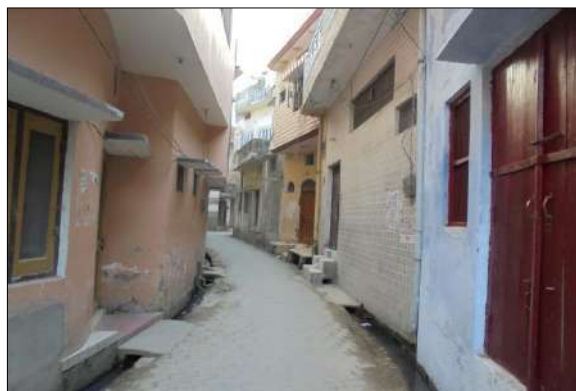
Figure 6-2: Housing in the Old City area
