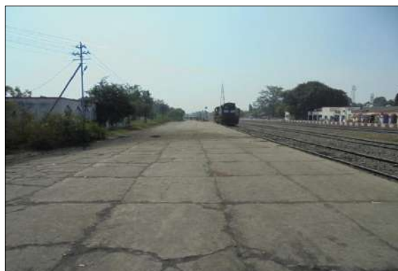
Figure 9-21: Goods Shed, Kashipur Junction Railway Station
